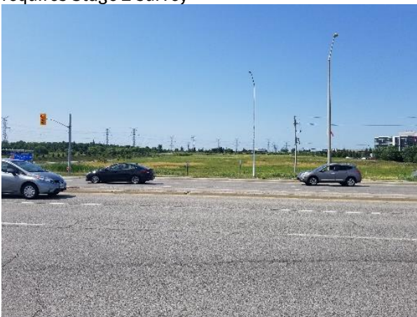
Plate 5: SW view Mississauga Rd and Hwy 407; Area beyond disturbed ROW requires Stage 2 survey
